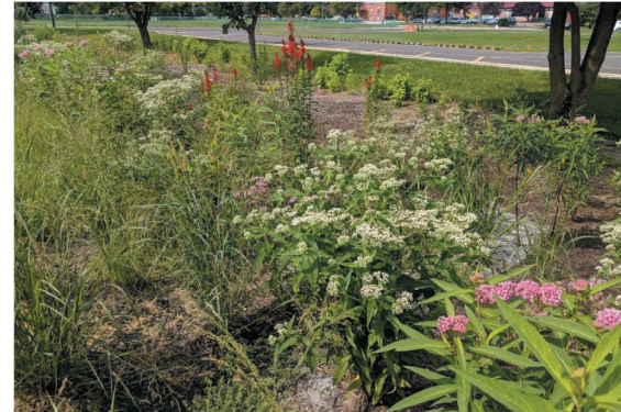
↑ Kenneth R. Olson Middle School in Tabernacle received funds from the South Jersey Landscape Makeover program to create this bioswale to capture rainwater and allow it to infiltrate the soil. This project was completed in May 2018.
