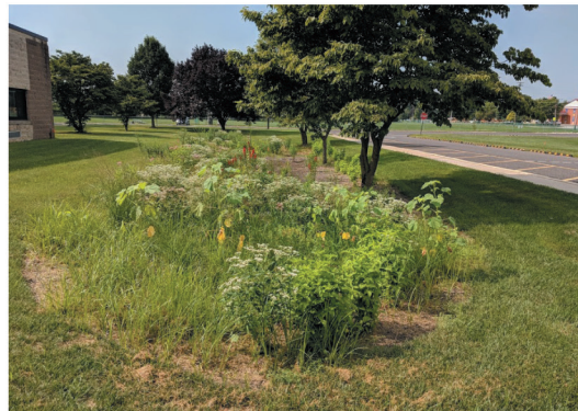
↑ Kenneth R. Olson Middle School in Tabernacle received funds from the South Jersey Landscape Makeover program to create this bioswale to capture rainwater and allow it to infiltrate the soil. This project was completed in May 2018.
