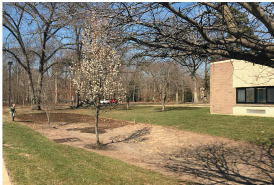
↑ Kenneth R. Olson Middle School in Tabernacle received funds from the South Jersey Landscape Makeover program to create this bioswale to capture rainwater and allow it to infiltrate the soil. This project was completed in May 2018.
